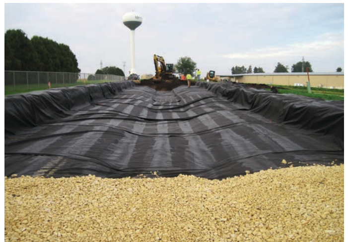
Bulldog Boulevard in Monona, Iowa, is prepped for permeable pavers in a green street project. Bulldog Boulevard was the second of two green street projects made possible through a sponsored project in conjunction with a State Revolving Fund. (Photo provided)
