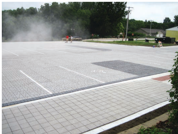
The permeable paver parking lot at the aquatic center in Monona, Iowa, has different colored pavers used as stripes between parking spaces and for distinguishing the handicapped spaces as well. Doing so cuts down on the cost of having to repaint those lines and symbols every couple of years. (Photo provided)
