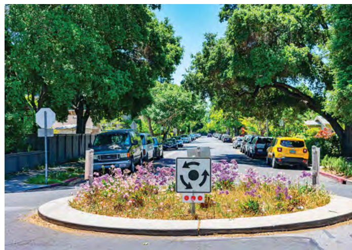
Traffic circles or roundabouts are also methods for traffic calming, reducing speeds and the volume of cut-through traffic. Pictured is a traffic circle in Palo Alto, Calif. (Michael Vi/Shutterstock.com)
