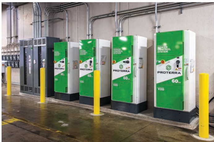
These are four charging stations for Proterra electric buses installed at the city of Wichita's transit garage. (Photo provided)
