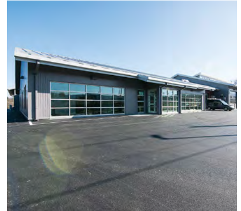
ABOVE: Effective communication between the city and its contractors kept the new public works operations center on schedule, saving money in the process. (Photo provided)
