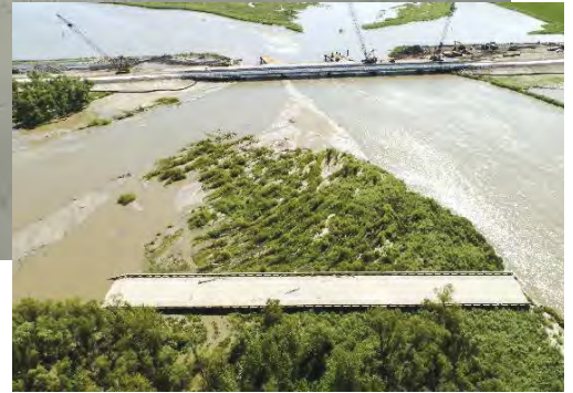
RIGHT: Highway 12's previous bridge deck was washed away in the flood near Niobrara, Neb. Behind it, construction work on the new bridge can be seen. (Photo provided)
