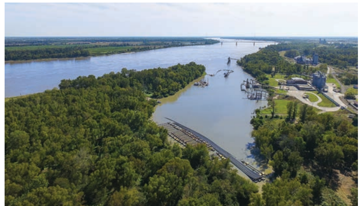
The Helena's Mississippi River Bridge connects Arkansas to Mississippi. Mayor members of the MRCTI have discovered they share a lot in common thanks to the Mississippi River, which creates similar concerns. (Photo provided)
