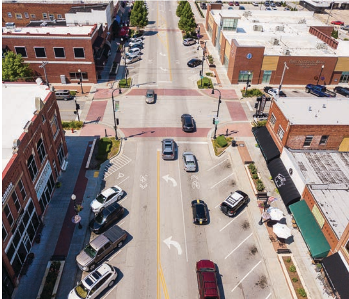
Road dieting was a major component of Broken Arrow’s Rose District streetscape project. Downtown was taken from four lanes to three lanes, slowing traffic and creating a more pedestrian-friendly environment. (Photo provided)
