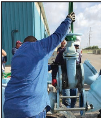
Spread outside flanges & remove old valve
