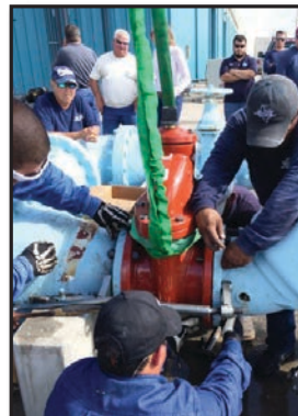
Reinstall new valve
