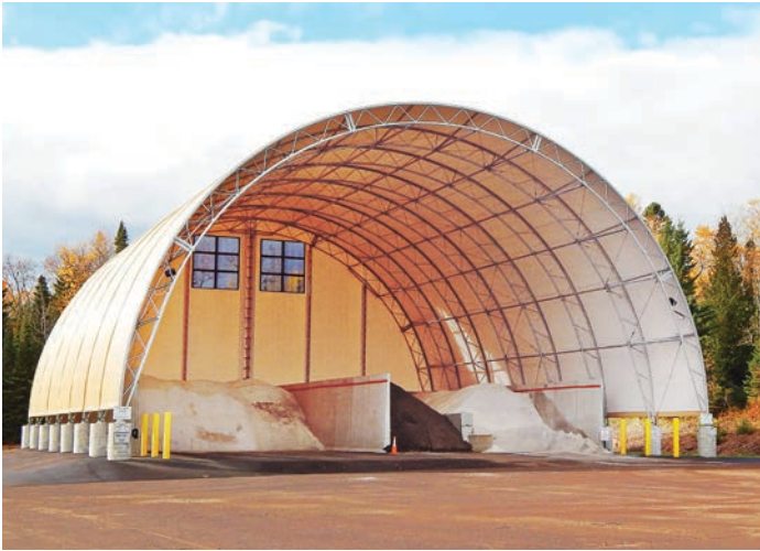
Shown is a municipal fabric building in northern Minnesota, which was designed and built by Greystone Construction. (Photo provided)
