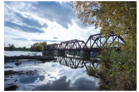
A bridge crosses over the River Raisin while wild fowl enjoy the water. (Photo provided)
