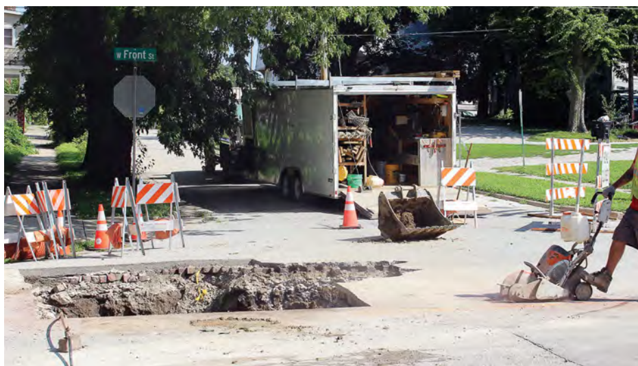
A public works employee cuts into the street as part of a sewer dig. (Photo provided)
