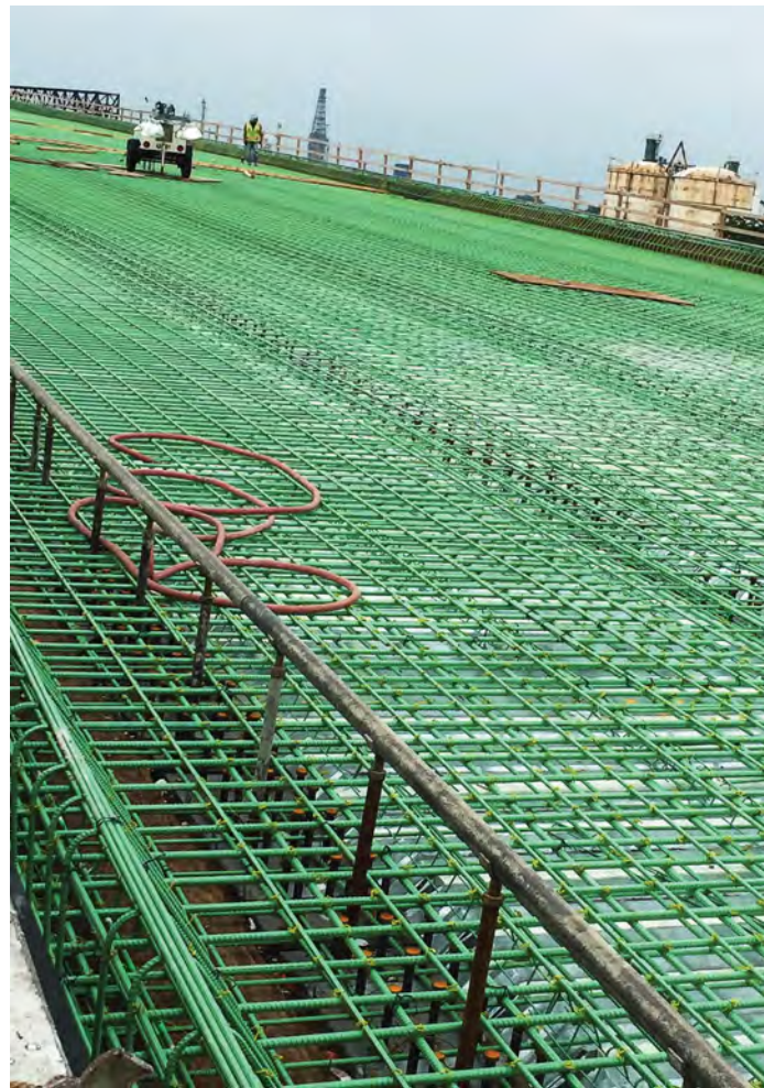
The Oakland County, Mich., I-75 Modernization project has seen the laying of miles of rebar, which has been made easier with the MAX Twintier RB441T, which improves worker safety while also preventing wire waste. (Photo provided)
