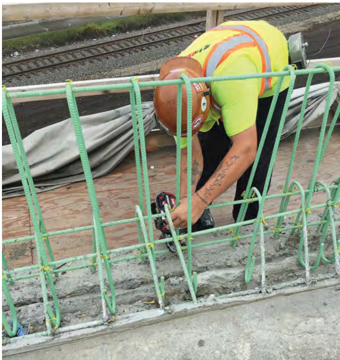
The tying of rebar predisposes ironworkers to the risk of developing musculoskeletal disorders to upper and lower extremities; MAX Twintier RB441T reduces this risk. (Photo provided)
