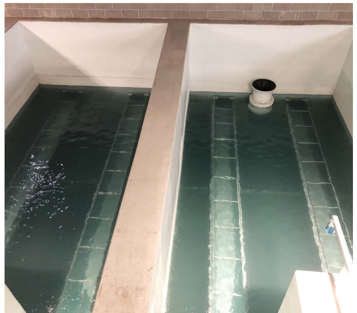
Unlike an in-home water softener, Morris' new system won't exchange sodium chloride for calcium; instead, it will remove calcium as lime sludge. (Photo provided)
