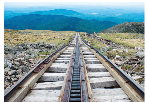
The mechanical structure of the cog railway ensures the train does not slip backward during its ascent or lurch forward on the way back down the mountain. (Shutterstock.com)
