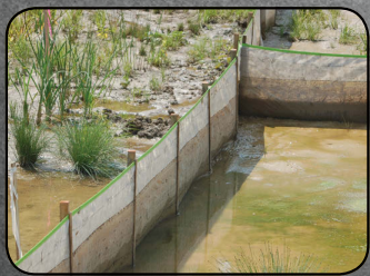
BSRF PRIORITY 1 SILT FENCE
