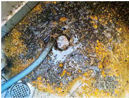
When fats, oil and grease build up in a sewer line it can lead to sewage backup and overflow into a yard, storm drain or street. Cleaning up and repairing this issue can result in hefty expenses and unfortunate effects to the environment. (Shutterstock.com)
