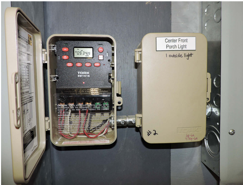
LEFT: While there are hundreds of facilities, Montgomery focused specifically on 75 buildings that made up $3 million of the $6 million annual utility cost. (Photo provided)
