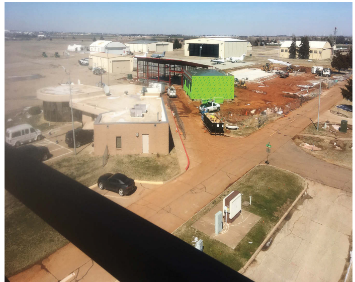
Pictured is construction work on the new terminal. (Photo provided)
