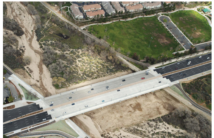
Santa Clarita Public Works Department widened the Newhall Ranch Road Bridge to include an additional lane in each direction and barriers in the middle of the road and to the sides for pedestrians. During this work, a bike trail and trail connection were added below the bridge. (Photo provided)
