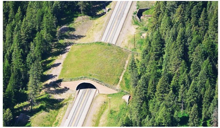
Wildlife overpass on US 93 south of Polson, Mont. (Photo provided by MDT, CSKT and WTI-MSU)
