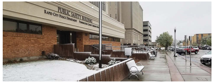
Pictured is the Rapid City Public Safety Building, which includes the Rapid City Police Department. The RCPD has been working through innovative programs to heal historic divisions in its community and attract more Native Americans to the police department. (Photo provided)
