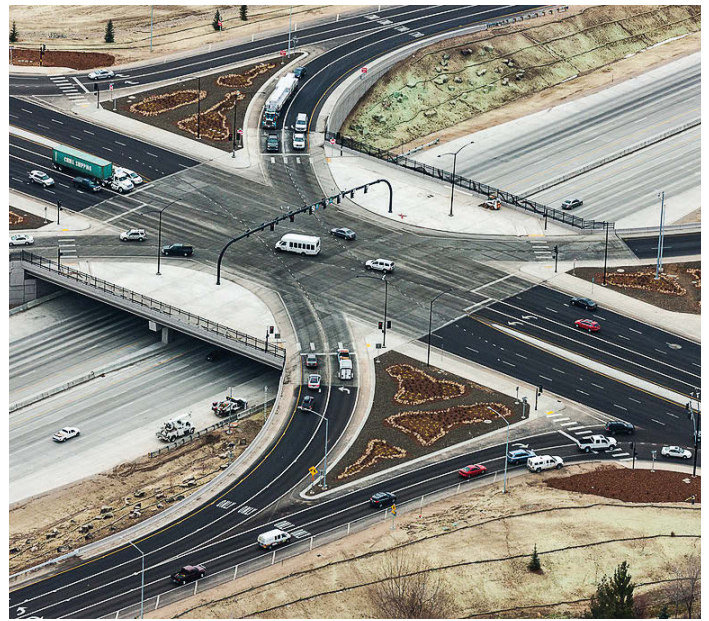
The widening of I-84 is just one of investments that the state of Idaho has put into the interstate over the years, especially as its usage is only expected to grow. Pictured is the I-84 Meridian Road Interchange in Meridian, Idaho, which was updated starting in 2012 to handle 284,000 vehicles per day as Meridian grows. (MeridianIdaho via English Wikimedia Commons; https://creativecommons.org/licenses/by-sa/4.0/deed.en )
