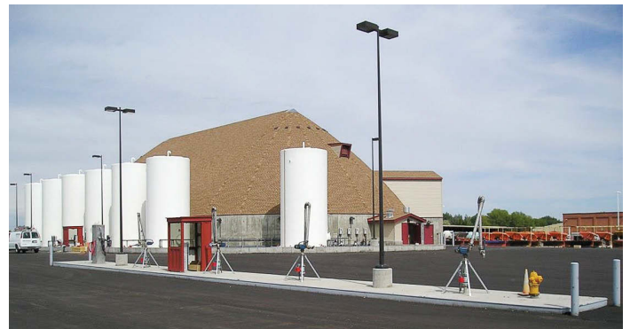
The material storage facility for snow removal was an approximately 10 months long project. The cost of the project after completion was $3.2 million. The facility holds 10,000 tons and the tanks have a 230,000-gallon capacity. (Photo provided by the city of Fort Collins, Colo.)
