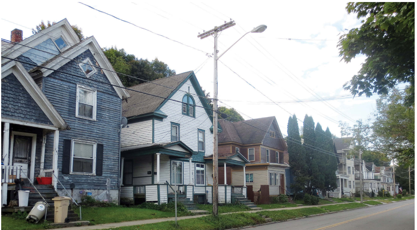
Originally, Ilion focused on converting 50 percent of the community to LED lighting and then decided to use 100 percent LED lights on its streets. Community feedback was extremely helpful for the village to determine how best to use the grant money. (Photo by Mitch Barrie; https://creativecommons.org/licenses/by-sa/2.0/ )
