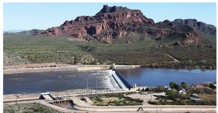
Granite Reef Diversion Dam diverts water from the Salt River into the canals to the north and south; this water is then delivered to water users within the Salt River Project. (Photo provided)
