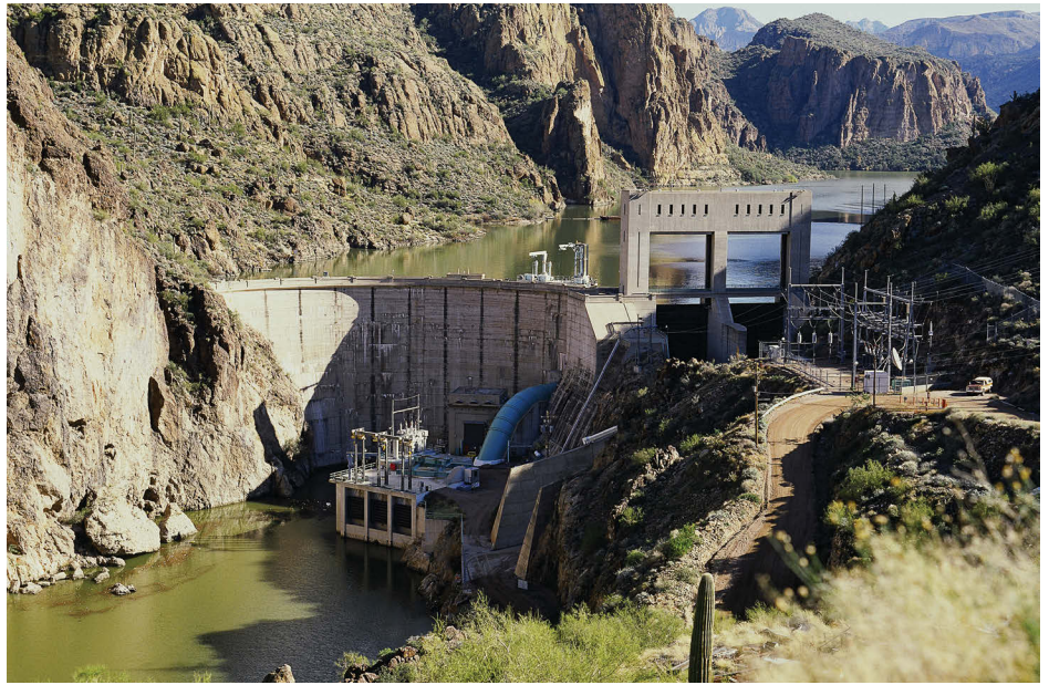
A part of the SRP, Mormon Flat Dam has two hydroelectric generating units; one is a conventional unit rated at 10,000 kW while the second is a pumped storage unit built in 1971 that is rated at 50,000 kW. (Photo provided)
