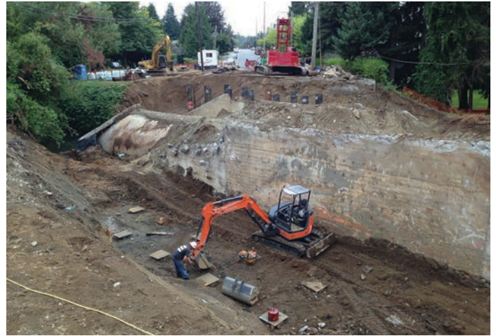
ABOVE & BELOW: An old culvert is cleared out in Lynden, Wash., allowing a new channel to be created. (Photo provided)
