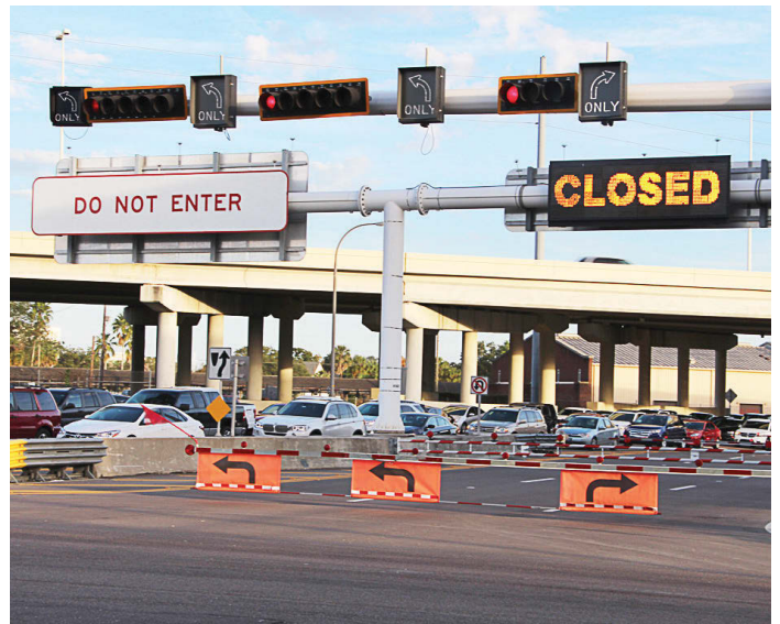
The downtown terminus of the Lee Roy Selmon Expressway Reversible Express Lanes is a potential entry point for wrong-way drivers. The Tampa Connected Vehicle Pilot will detect and warn wrong-way drivers before they get on the expressway. Other drivers on the REL will also receive a warning if a wrong-way driver is approaching. (Photo provided)
