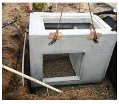
StormTree, with its compact size and open sides, provides ease of installation and cost management. Often the only piece of equipment needed for installation is a mini excavator. (Photo provided)
