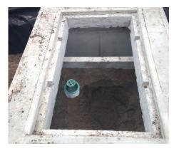
Pictured is the interior of the precast frame. StormTree's frame is open bottom and open sided with a filter media area allowing for unrestricted tree root growth. (Photo provided)
