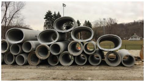
Replacing more than 1,600 linear feet of cement-lined, ductile iron water main pipes as well as 900-plus feet of connection pipes of varying diameter was a major part of the infrastructure and streetscape plan. They were replaced with 24-inch reinforced concrete piping as well as a new 915-foot twin DIP. (Photo provided)
