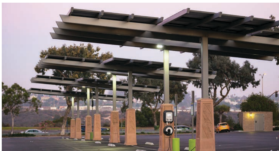
EV stations have a 10-year or more life span and are pretty low maintenance. With a networked station, there are over the air upgrades that occur throughout the life of that station. Pictured is a solar-powered EV station in a public parking lot in San Diego, Calif. (Joshua Rainey Photography/Shutterstock.com)
