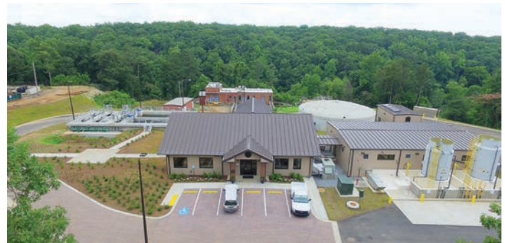
Roswell’s new water plant has the treatment capacity of 3.2 million gallons per day. The project required a lot of creative thinking to work within a small budget. (Photo provided)
