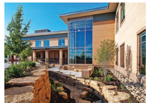
Fitchburg installed 362 kW of solar photovoltaic panels on the roofs of the library, city hall, public works maintenance facility and a fire station in 2017. Pictured is Fitchburg City Hall's North Reading Garden. (Photo provided)
