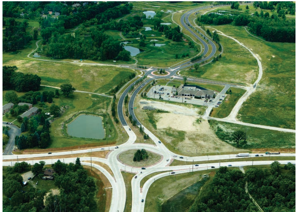
Commercial semi-trailer trucks routinely navigate the M5 roundabout in Oakland County, Mich. The roundabout is designed to compensate for the trucks' wider turn radiuses. (Photo provided)
