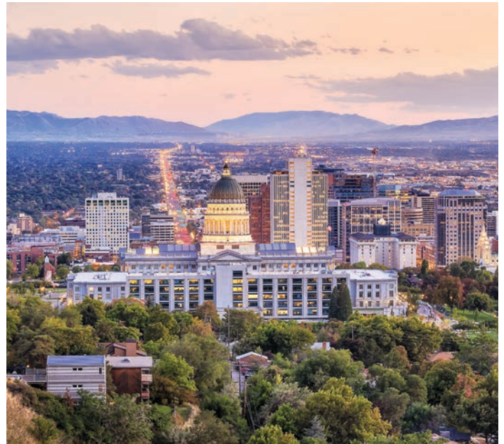
Salt Lake City, Utah, has installed solar panels on 14 separate facilities as part of its goal to power its government operations, and ultimately the whole community, with 100 percent renewable energy. (Shutterstock.com)
