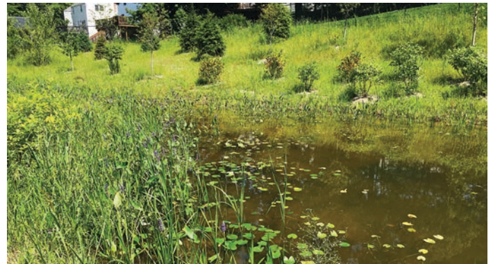
This is the created wetland in Albany, N.Y., in August 2017—just six months after construction was completed and four months after plantings. Commissioner Joe Coffey remarked that already at this point the wetland looked as if it had always been there. (Photo provided)
