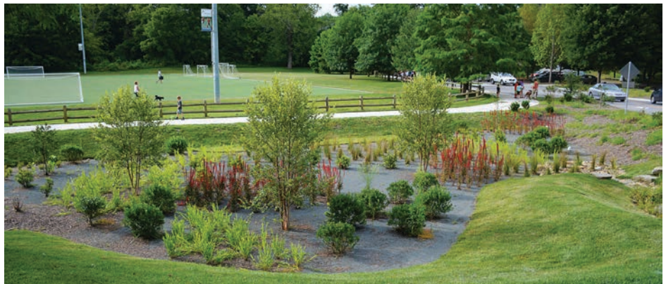
This bioretention pond at Azalea Road in Asheville has more plantings than a normal retention pond for aesthetics and to help treat the stormwater. Stormwater Services Manager McCray Coates said any time the city does roadwork now they are incorporating stormwater features like porous pavers, biocells, etc. (Photo provided)
