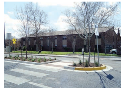
Pedestrian safety islands are another design that cities are choosing to install. Small updates can also improve safety, such as clearly painting crosswalks and checking that both street signals and walk/don't walk signs are operational. (Photo provided by National Association of City Transportation Officials)
