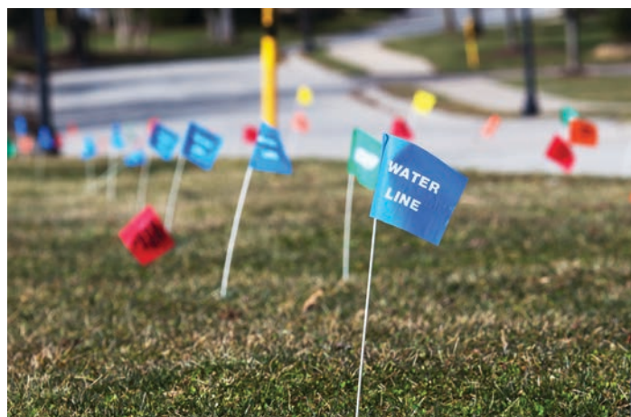
ABOVE: Marking utility lines above ground isn't always enough. Sometimes the different lines can be of the same build, which doesn't help the contractor. Every available piece of information should be accessible to avoid any delays or other issues. (Shutterstock.com)
