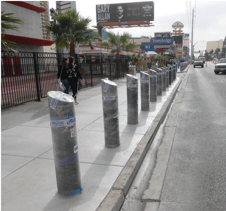
Following a driver driving onto the sidewalk on the Las Vegas Strip, Clark County, Nev., installed physical barriers to prevent any vehicles from accessing sidewalks on the strip. (Photo provided)
