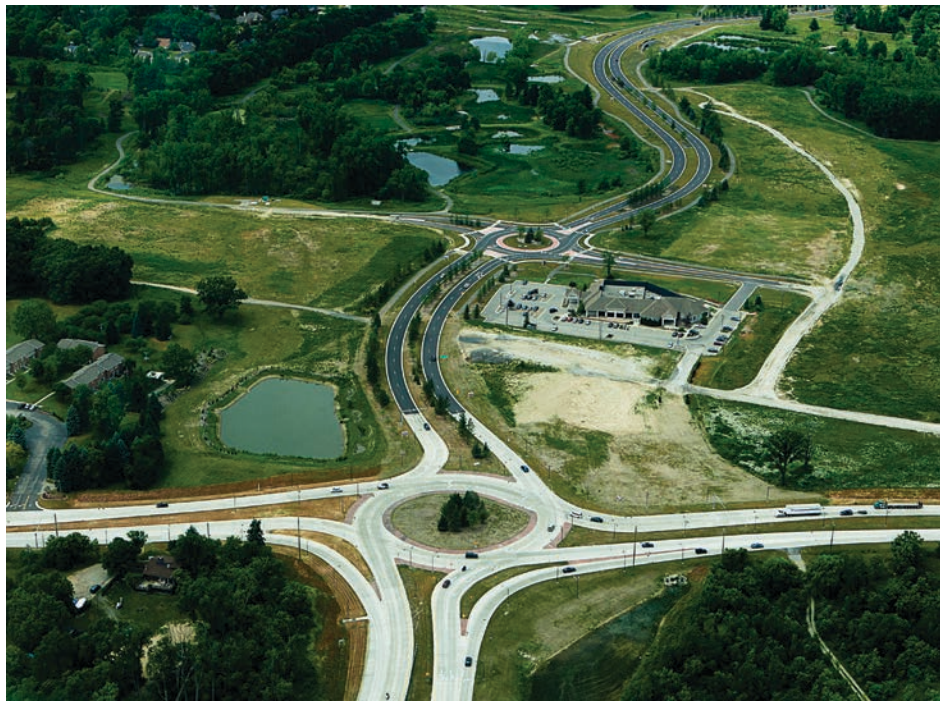
Pictured is the M-5 and Martin Parkway roundabout in Oakland County, Mich. (Photo provided by Road Commission for Oakland County)
