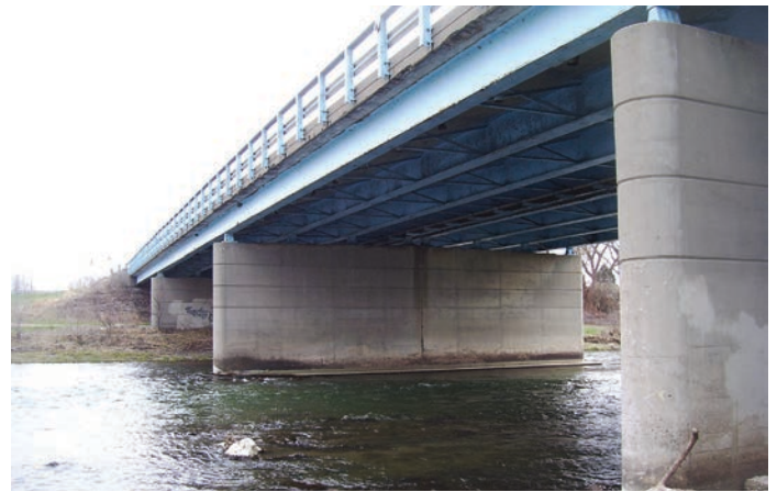
ABOVE: Pictured is the Harshman Road Bridge in 2011. Its deck had been falling apart while cracks had appeared in the pier and abutment walls. Erosion also posed a concern. (Photo provided)
