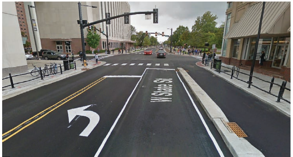
Pictured is the new two-way State Street in West Lafayette going toward Purdue University’s campus. With State Street being the main roadway going through campus, the change to a two-way creates a more welcoming impression. (Photo via Google Maps)
