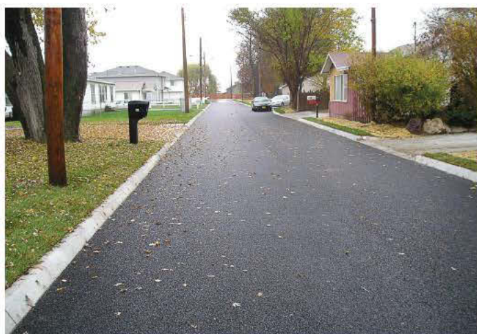
This "after" photo shows a recently installed porous asphalt road in the East Manawa neighborhood of Council Bluffs. The pores in the asphalt are visible in the photo. Not only does the porous asphalt help with drainage, it's been making cleaning the streets of ice and snow easier, plus it improves the overall look of the neighborhood. (Photo provided)
