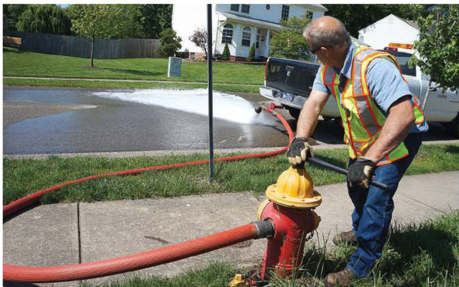
Local governments often have more of an impact on daily lives of citizens, through maintaining necessary infrastructure. Pictured, a Cranberry Township employee flushes a fire hydrant. (Photo provided)
