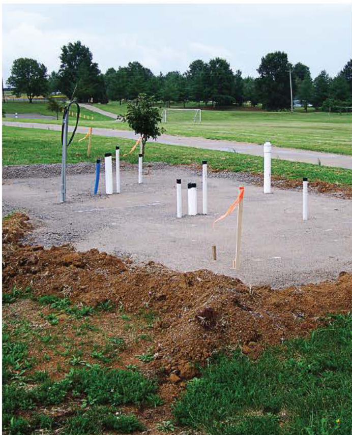
Sewer pipes, water lines and electrical lines needed to be installed prior to the installation of the prefabricated restrooms. The city of Perryville, Mo., is installing these restrooms to cut down on instances of vandalism. (Photo by Keith Riney)
