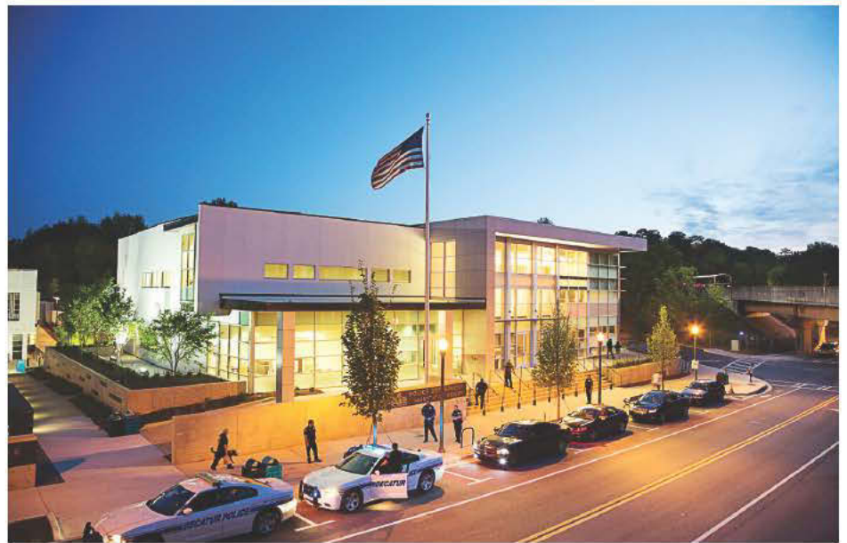
Decatur adopted a policy where every city-owned building over 5,000 square feet has to be certified as a Leader in Energy and Environmental Design by the U.S. Green Building Council. Pictured is Decatur's Beacon Municipal Center (Photo provided)
