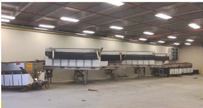
Due to the expansion, the city of Farmington Hills has more indoor storage for equipment like these salt spreaders. Indoor storage gives equipment longer life. (Photo provided)
