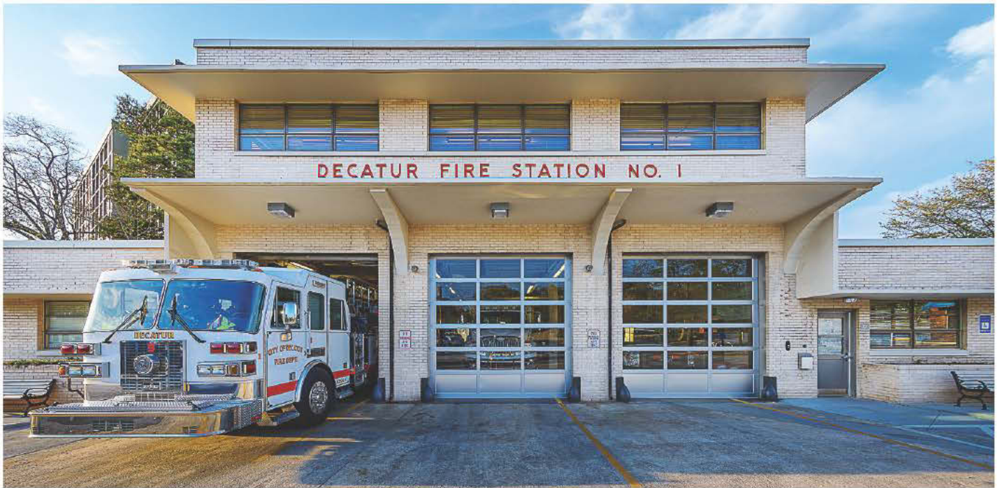
Decatur Fire Station No. 1 received a complete renovation and expansion—a project that achieved LEED Platinum certification. (Photo provided)
