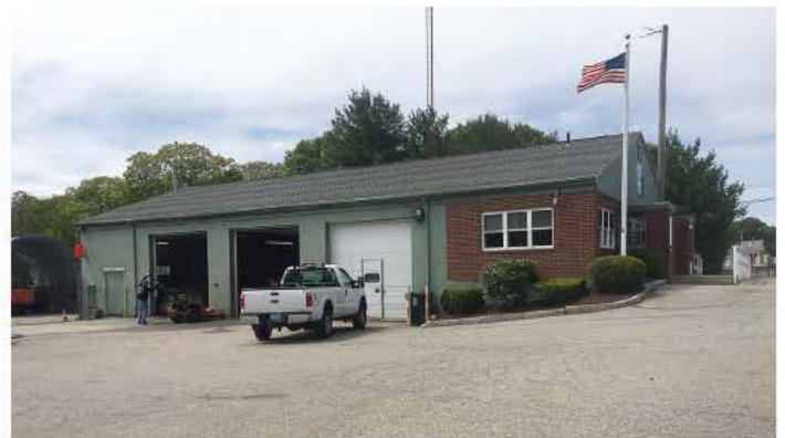
Swansea's highway department is in great need of a new garage for its vehicles, making the abandoned Sears' fully operational car facility appealing. (Photo provided)
