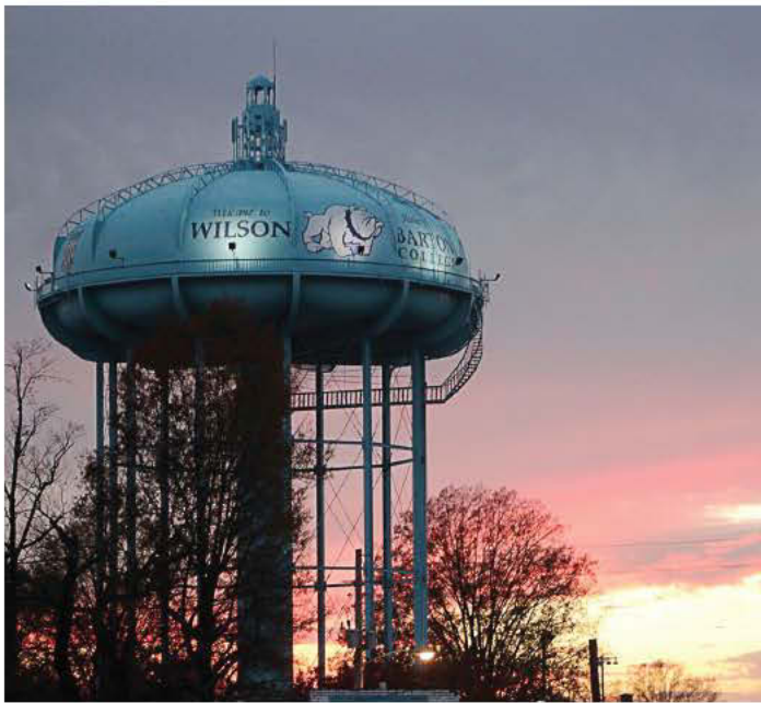
When Wilson made the transfer to smart meters in hot weather, the town's staff worked diligently with help from water, Gatorade and popsicles to keep them hydrated. Wilson's citizens are very appreciative for all that the workers do. (Photo provided)
