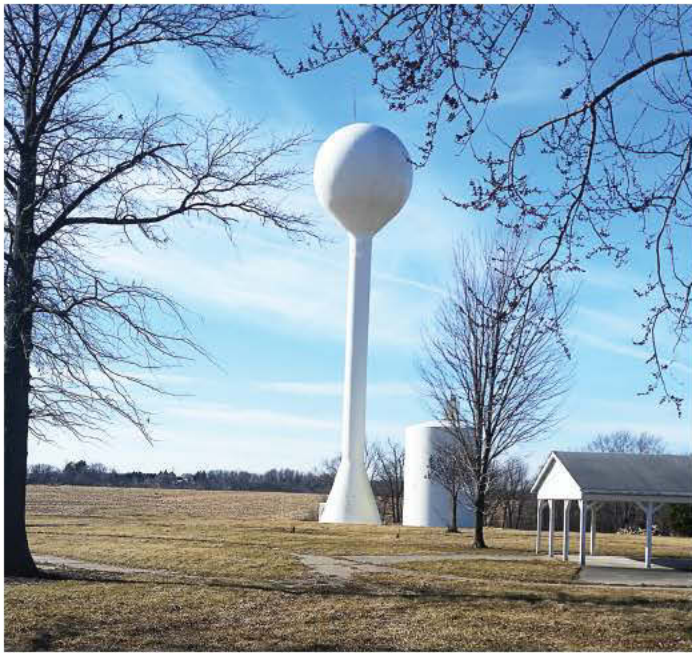
Rock Island County is set to dedicate two surplus water tanks — a 150,000 elevated spheroid and 100,000-gallon steel ground storage — to Moline as part of a regional effort to encourage development within the Illinois Quad Cities. (Photo provided)
