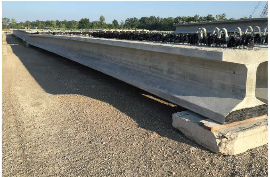
The bulb T-beams, along with the carbon fiber reinforcement, are expected to reduce concrete cracking, deterioration and corrosion that is typical in traditional steel reinforced bridges. (Photo provided)
