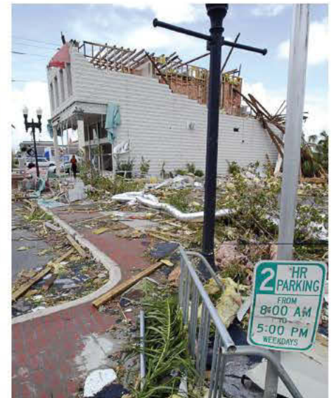
Pictured is Marion Avenue and a glimpse of the damage left behind by Hurricane Charley. (Photo provided by Punta Gorda)
