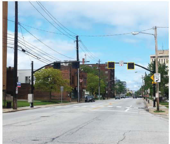
A HAWK system is designed to stop traffic only as needed when pedestrians are present at the crosswalk. Pictured is the signal at Manor Park and Detroit Avenues. The silver box on the left is the signal controller cabinet to operate the signal. (Photo provided by Lakewood, Ohio)
