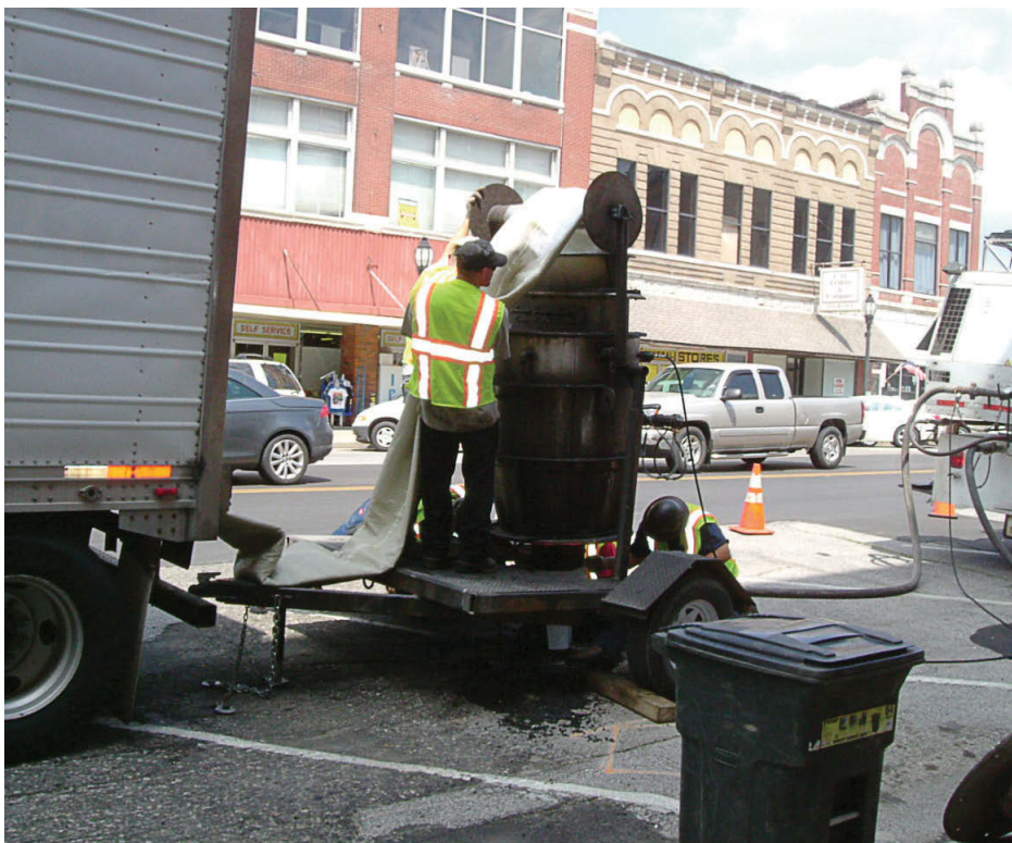
ABOVE LEFT: While installing new water lines in Henderson, workers also addressed sewers that already took stormwater, lining them with in situ form. (Photo provided)
