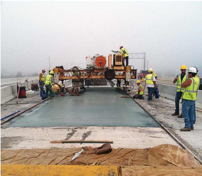
Contractors hand-level the concrete as they complete the bridge deck overlay on the I-69/SR 1 project in Fort Wayne, Ind. (Photo provided by INDOT)
