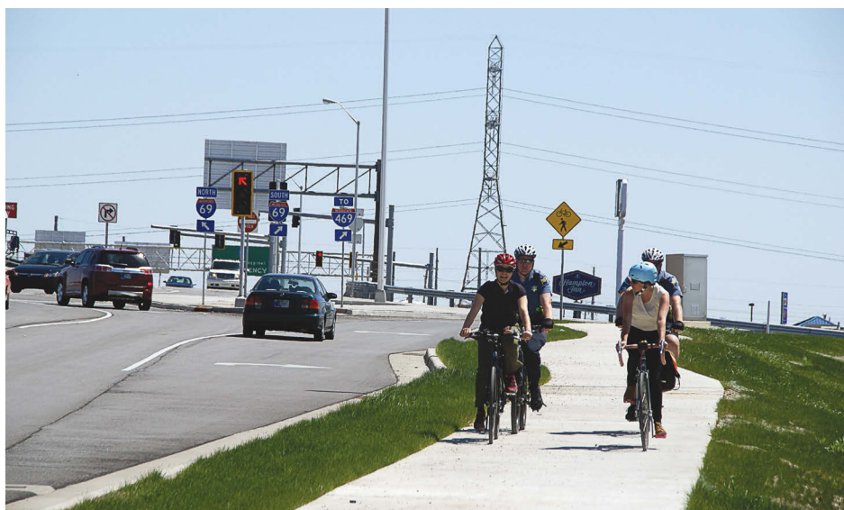
RIGHT: Fort Wayne's diverging diamond interchange has streamlined traffic, cutting down commute times. In general DDIs have been shown to decrease overall accidents by more than 55 percent. (Photo provided by INDOT)
