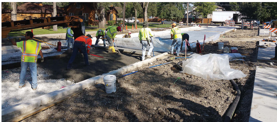
Pervious concrete allows water to seep through its open pores and be collected in a base below to be reabsorbed into the ground or evaporated. (Photo provided)
