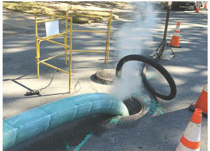
Cured-in-place pipe technology utilizes a felt tube saturated with resin, which is inserted into a weak pipe via manhole access. Once this liner is installed and in place, applied pressure—using air or water—swells the liner to fit nicely within the confines of the old pipe. (Photo courtesy David Poe/Pine Bluff Wastewater Utility)
