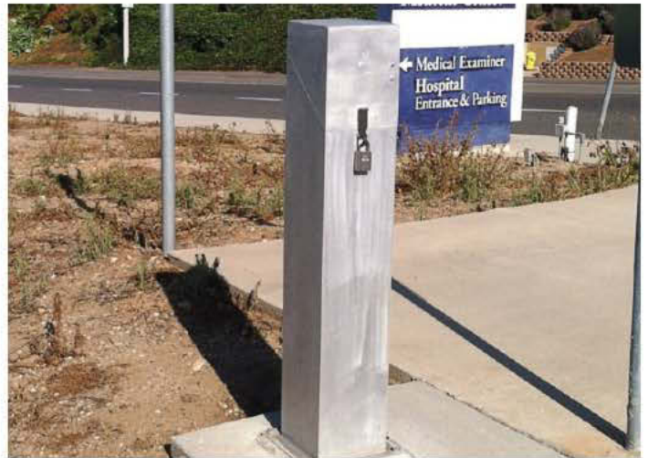
A water sampling station in Ventura County, Calif., is sealed to protect it from damage, tampering and contamination. (Photo provided)
