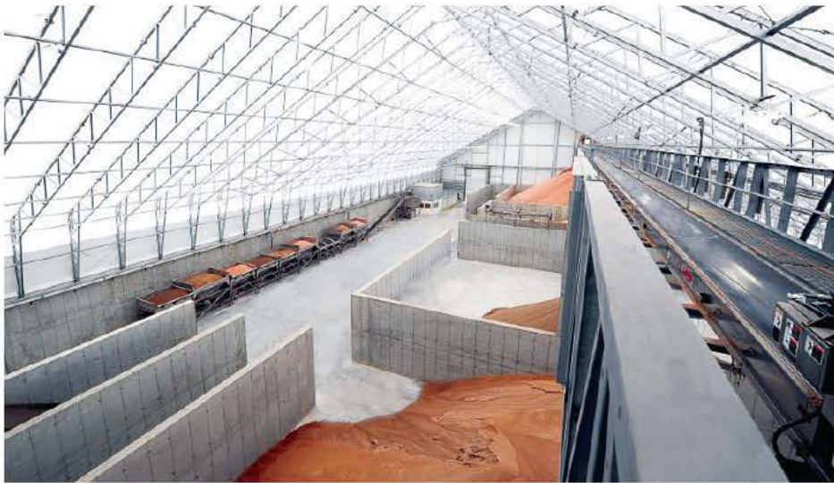
Temporary structures are popular options for storing commodities like sand and salt; this prevents runoff that could create an environmental disaster. (Photo provided by Calhoun)
