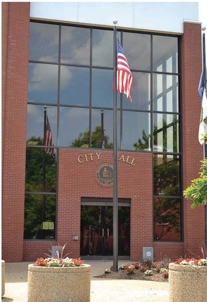
ABOVE LEFT: The entranceway to Manassas City Hall is monitored for any possible tripping hazards. (Photo provided)
