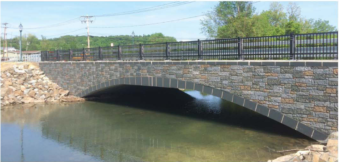
The arch on the completed Elk Drive Bridge is a Bebo system by Contech Engineered Solutions. The headwalls were also precast; the stone pattern was stained in the field to give it the look of natural stone. (Photo provided)
