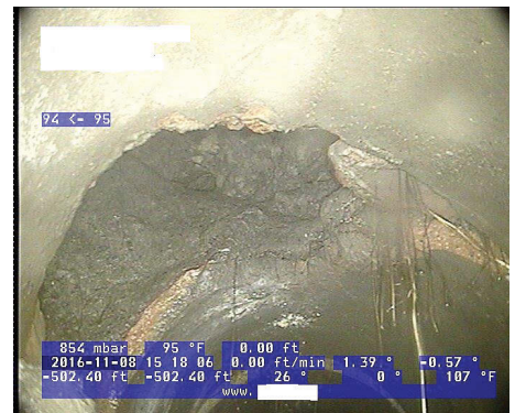
Pictured is the interior of a sanitary sewer main as it is checked for a pipe failure (Photo provided by Oskaloosa Water and Wastewater Department)
