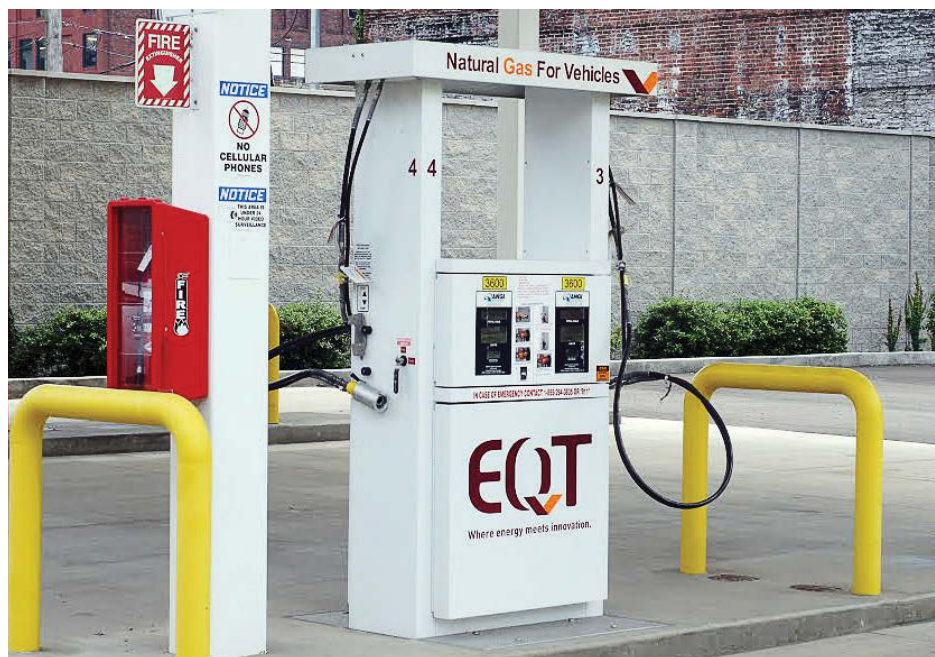
CNG is safer when fueling than gasoline or diesel since it uses a closed system, meaning no fumes are emanating from the gas tank. (Photo provided by National Alternative Fuels Training Consortium)
