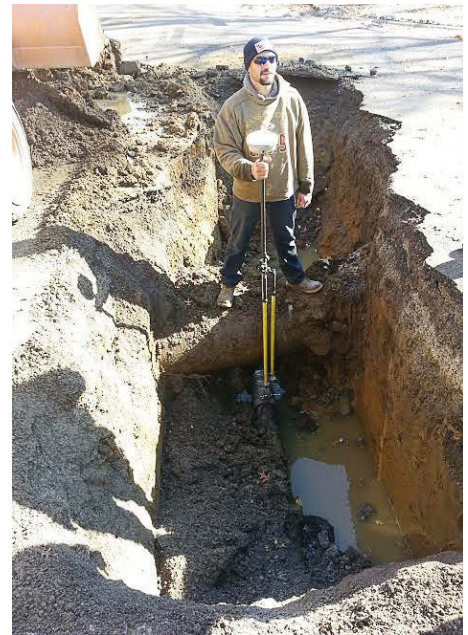
A worker installs the new section of water main and new fire hydrant. (Photo provided by Oskaloosa Water and Wastewater Department)
