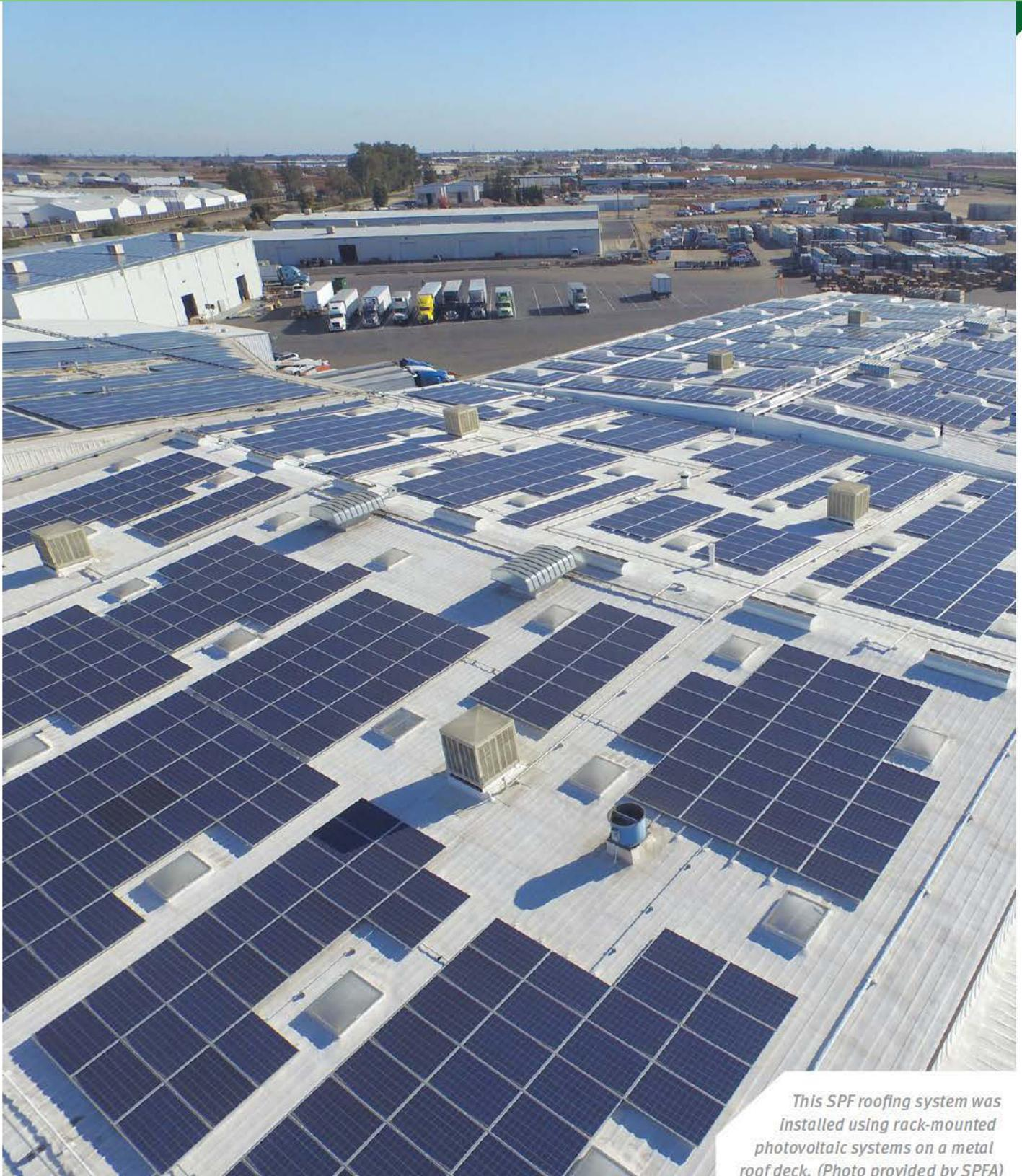
*This SPF roofing system was installed using rack-mounted photovoltaic systems on a metal roof deck. (Photo provided by SPFA)*
