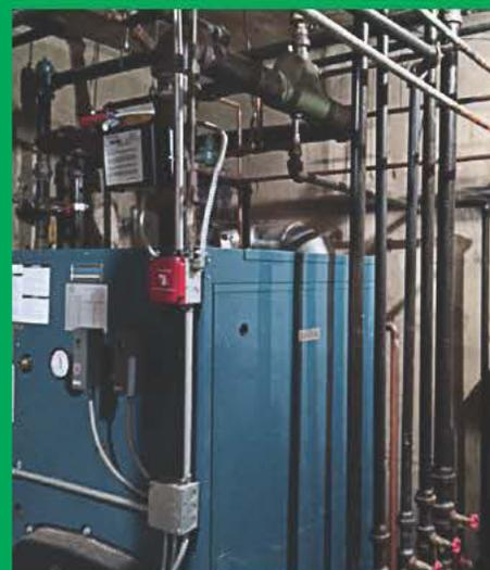
As a part of its retrofitting, East Rockaway added pipe insulation in its boiler room. Pictured above is the before; below is the after. (Photo provided by Johnson Controls)
