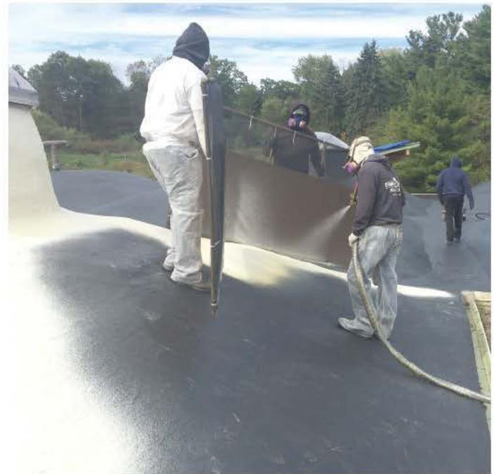
*Pictured is a spray polyurethane foam roofing system being applied over a primed commercial roof. (Photo provided by SPFA)*
