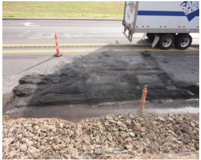
The loose millings were removed.
