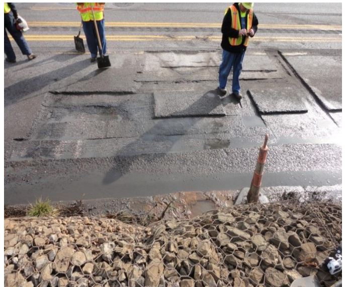
Sections of hotmix were left in place to use as a control material and to compare performance to UPM. Looking closely you can see the water seeping up through the HMA into the recently milled areas.
