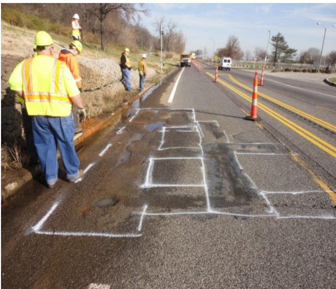
After setting up a work zone, the area was marked. Using a milling head mounted to a skid steer loader, 1-1/2 to 2 inches was milled from the road surface.
