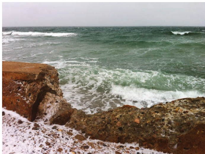
Prior to the North Bluff renourishment project, an old seawall had failed due to erosion. (Photo provided)
