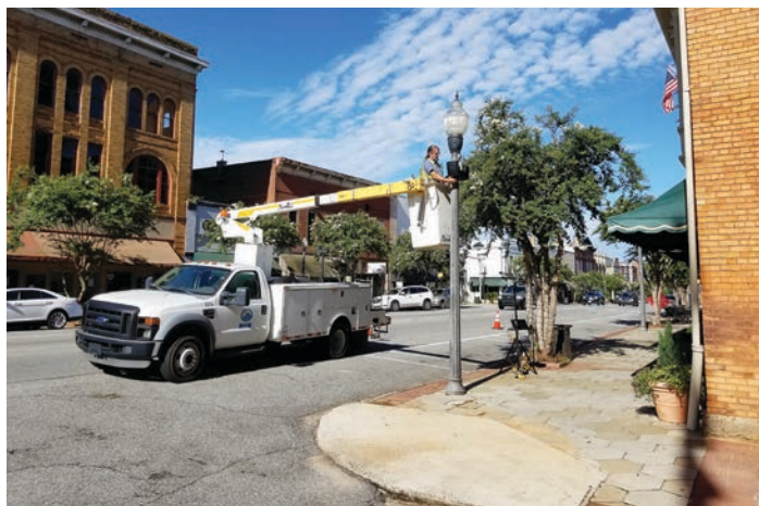
A public works employee uses a bucket truck to install a StreetSounds pole-mounted speaker unit. (Photo provided)
