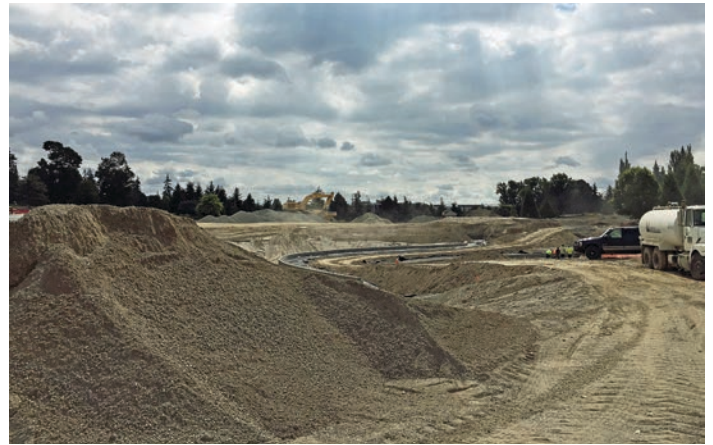
Retaining wall construction at ponds A and B is shown at the Legion Memorial golf course. Considering design specifics for the detention ponds, certain criteria needed to be met regarding side slopes, the access ramp grade, access road and ramp width, pond walls and using a safety bench in lieu of a fence. (Photo provided)
