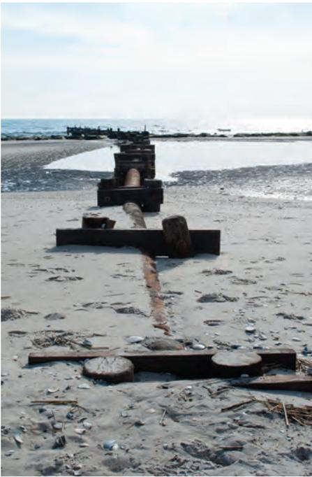
*Myrtle Beach has installed deepwater ocean outfalls similar to this one in Cape May, N.J. This outfall tube was exposed in 2010 after a severe storm. Other cities along the East Coast have turned to outfalls to prevent or reduce flooding, with Myrtle Beach launching its outfalls after learning about their use in Virginia. (Photo by Michael Medina-Latorre/FEMA)*
