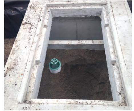
*Pictured is the interior of the precast frame. StormTree’s frame is open bottom and open sided with a filter media area allowing for unrestricted tree root growth. (Photo provided)*
