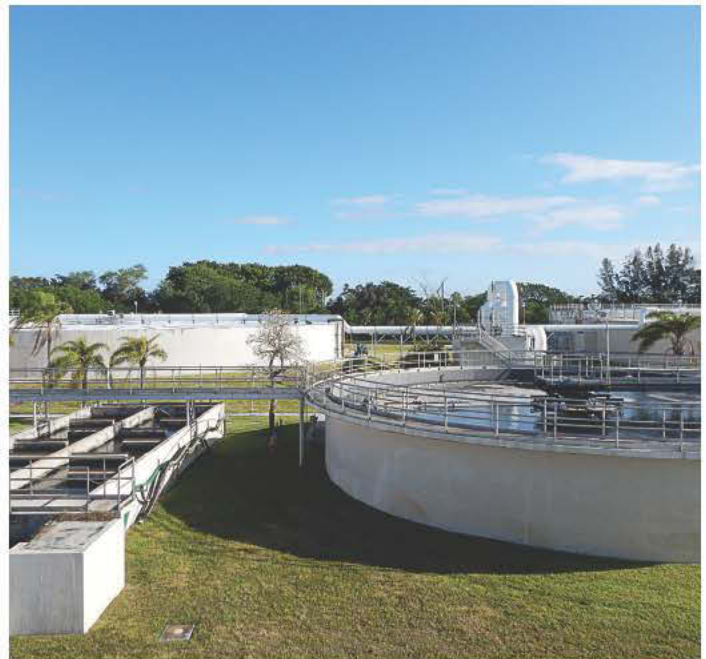
Wellington, Fla.'s, water reclamation facility is located on a very small property, 25 acres, and has a treatment capacity of 6.5 million gallons per day. (Photo provided by Bryan J. Gayoso)
