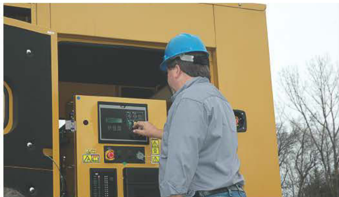
As part of routine testing, Hinckley Wastewater Treatment Plant personnel will run the genset under no load once a week for at least an hour. Once a month, staff transfers the generator load to run the plant anywhere from one to four hours. (Photo provided)
