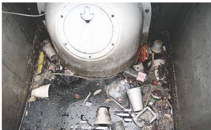
A 30F Snout in Myrtle Beach, S.C., traps trash, debris and oils. (Photo provided)
