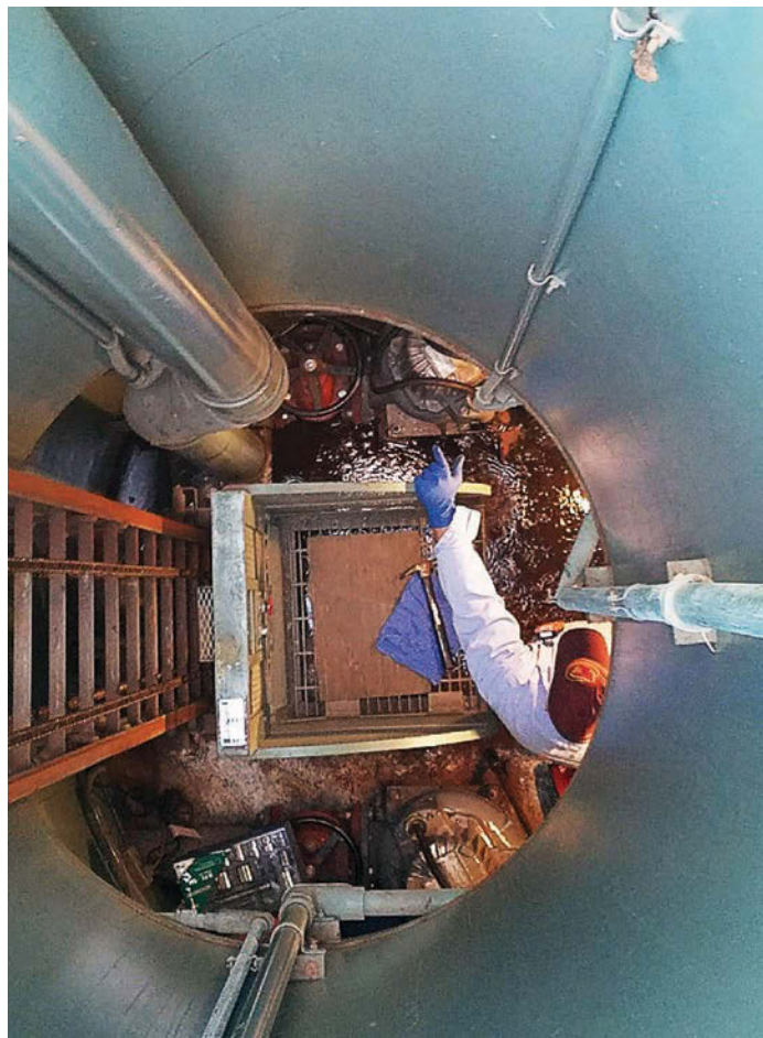
Des Moines workers complete a pump station valve replacement. (Photo provided)
