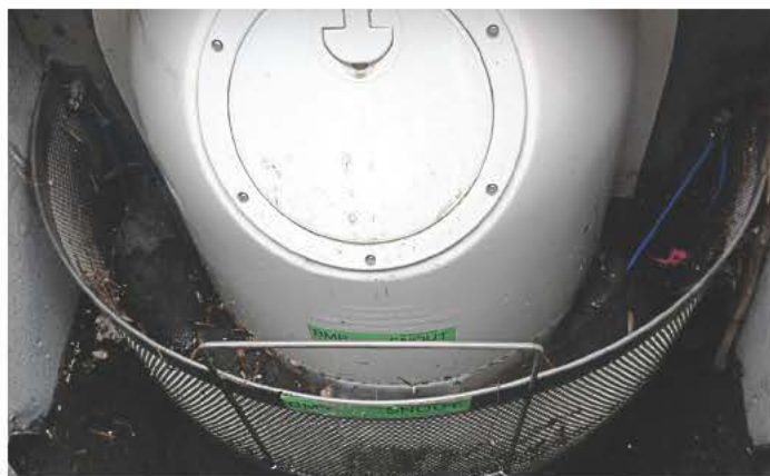
Pictured is a Snout, Bio-Skirt and stainless TrashScreen in North Myrtle Beach, S.C. (Photo provided)
