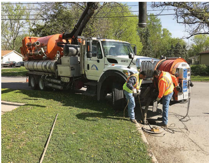
Public works employees continue sewer cleaning using pipe jetting. (Photo provided)
